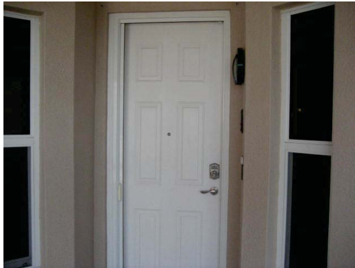
Reinforced masonry exterior walls | Hurricane Impact Windows and Doors
